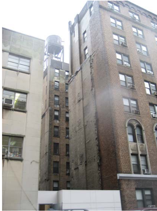
Easterly Wall & Courtyard of 18 West 70 th Street
